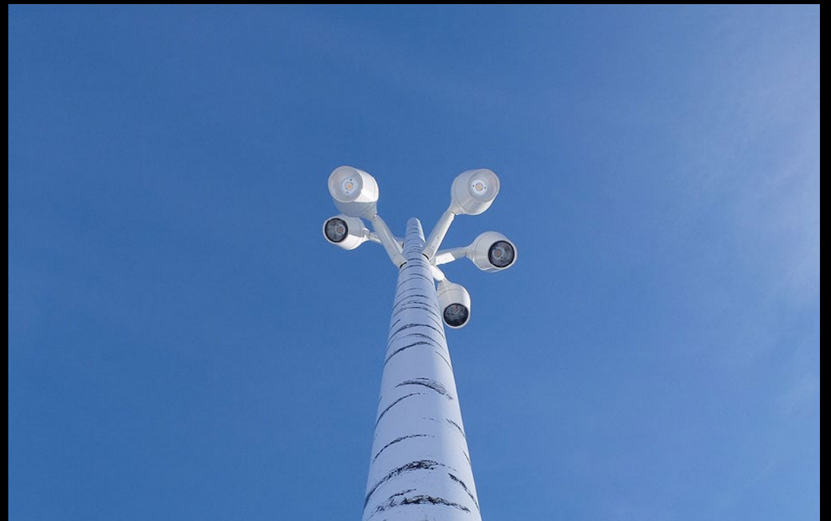
Mâts Design 8 m — Lerum, Suède Lighting Column Design 8 m — Lerum, Sweden
